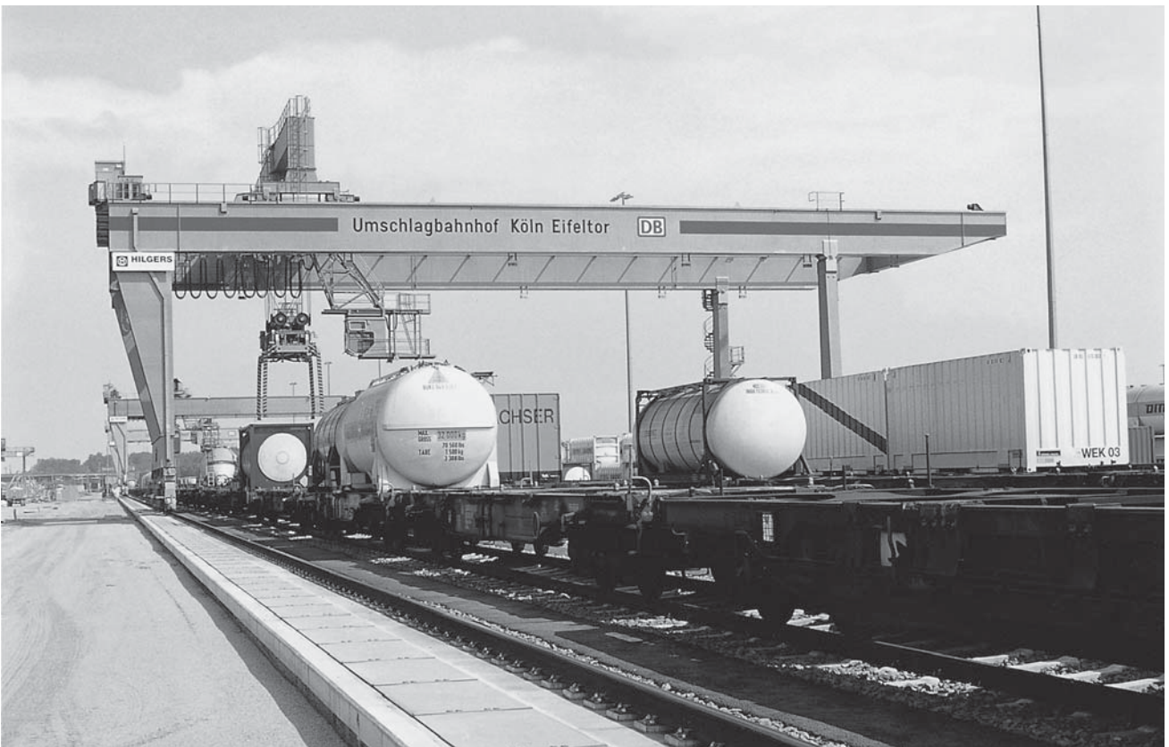
VAHLE-EID conductor trench for container terminal
